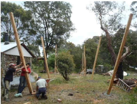
Volunteers assisting with erecting the main posts for Quil's enclosure in 2014
